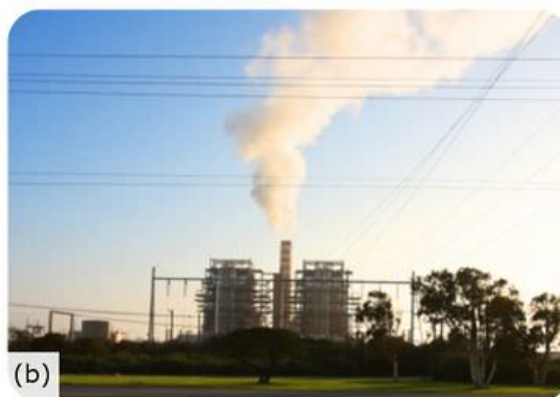
(b) A small coal-fired power plant.
