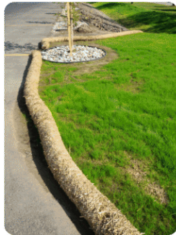
Hold soil in place at construction sites.
