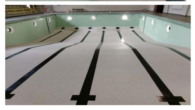
In November 2017 Edison's pool underwent a deep cleaning. Elite Pool Tile Cleaning had a large task of cleaning and repairing tiles in the pool. First the pool had been drained and then the cleaning began. Tiles were first bead blasted, then hand scrubbed. Tiles were repaired or replaced and lane markers and deck depth markers were painted. Project is still underway and should be completed and pool filled by February 2018. So far contractor's team has worked approximately 800 labor hours.
